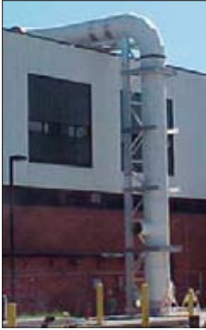
Odor control duct systems for water treatment
