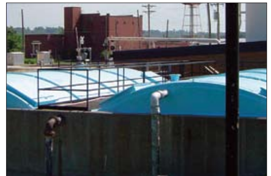
Tank covers, designed for snow and live loads
