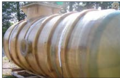
Underground storage tank
