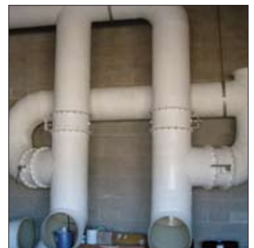
Prefabricated corrosion resistant duct system for water plant chlorine room
