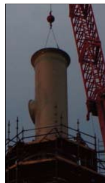
Stack liner, 6' diameter x 40' section of 200' stack
