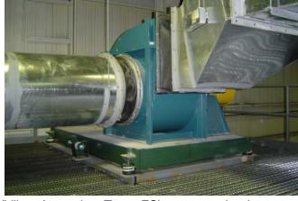
A Concrete Inertia Base (Vibro-Acoustics model CIB) provides a rigid platform to hold various types of equipment, such as base-mounted pumps, air compressors and fans. By lowering the equipment's center of gravity and reducing the amplitude of vibration, the CIB controls the vibration transmission into the structure.
