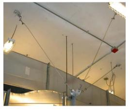
Society of Civil Engineers' document, ASCE-7-05 to determine the design forces used in selecting appropriate sway bracing and seismic restraints. Bracket size, cable diameter and anchor bolts must be selected correctly to resist the expected forces. Other guidelines are published by SMACNA, ASHRAE, and FEMA.
