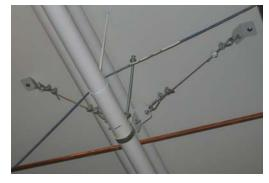
Examples of cable restraint sway bracing on ductwork and pipe (Vibro-Acoustics models SRK-400, SRK-800, SRK-
