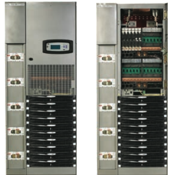
LPS, -48VDC, 10,000A Modular Power Plant
