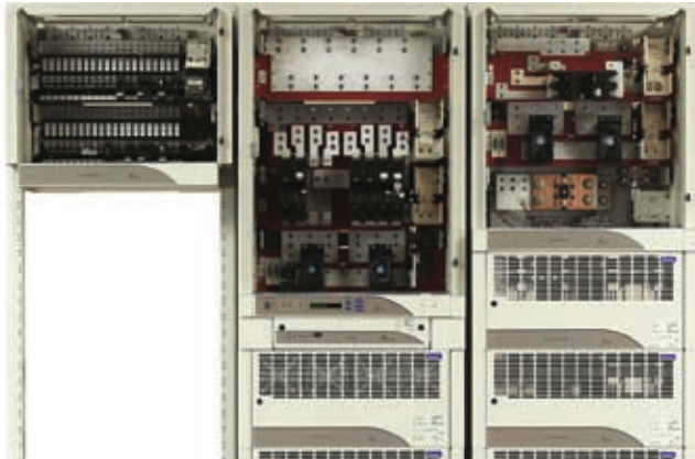
Modular Distribution Cabinets
