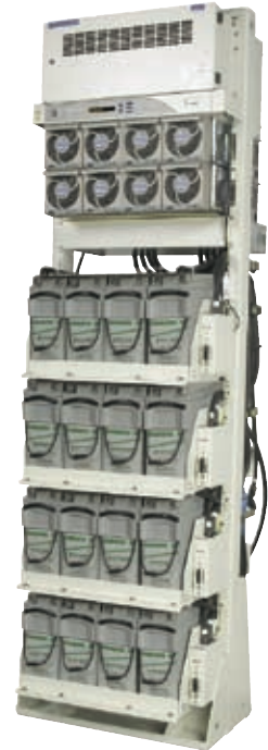
-48VDC 500 amp VPS with Battery Trays
