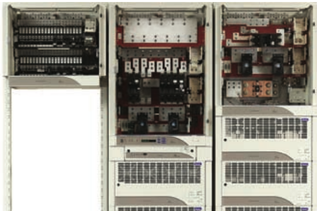
Modular Distribution Cabinets
