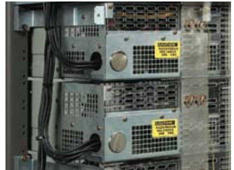
Bottom AC Wireway Input (cover removed)
