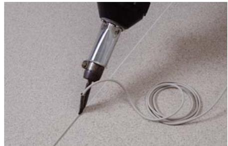
Weld rod seam
