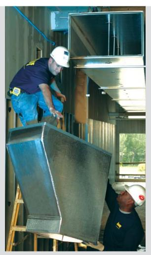
**Easy Handling:** KoolDuct panels are 15% of the weight of insulated sheet metal ductwork, making fabrication, transport and installation fast and easy.
