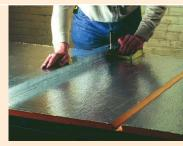
Glue and fold panels at grooves to form air duct segment.
