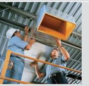
Knauf Air Duct Board-AGM has a mat-faced airstream surface and a Foil-Scrim-Kraft (FSK) facing on the outside.
