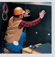
Knauf Rigid Plenum Liner offers an optimal combination of efficient sound absorption, thermal conductivity and minimal air surface friction.
