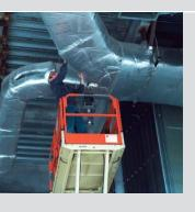
Knauf Friendly Feel Duct Wrap for cooling, heating or dual temperature service.
