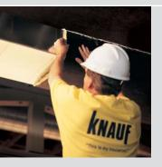
Knauf Duct Wrap with Black PSK facing is a desirable solution for exposed ductwork eliminates the need to paint.
