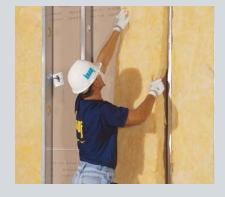
· Knauf QuietTherm Insulation's excellent acoustical properties reduce sound transmission when properly installed in metal frame buildings.
