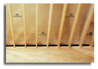
On a hot summer day, attics with Thermostat® OSB Radiant Barrier Roof Sheathing can stay up to 30° cooler than attics with standard sheathing
