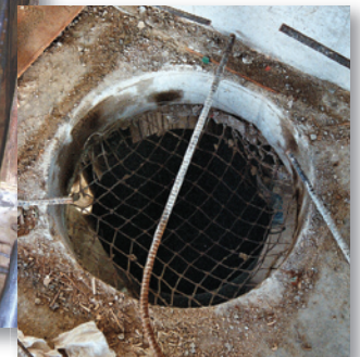
Pour-In-Place Netting System After Installation v
