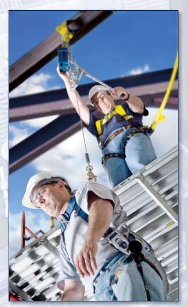
Provides Quick, Efficient, and Safe Rescue for a Worker Who Has Fallen While Connected to a Cable Self Retracting Lifeline (SRL)
