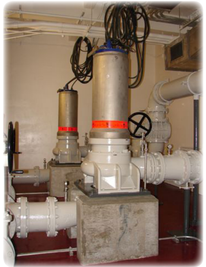
Three (3) 12" discharge, 161 hp closed-loop cooling dry-pit pumps with stainless steel Jacket in existing pumping station.
