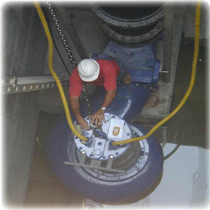
Two (2) large 24" discharge, 148 hp Submersible Pumps with stainless steel cooling jacket on KSB guide rail system for an effluent waste water treatment pumping station.
