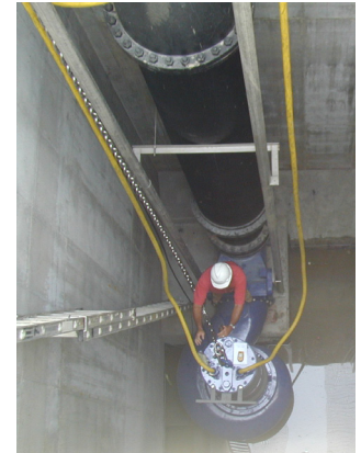
Two (2) 148 hp Submersible Pumps with cooling jacket.
