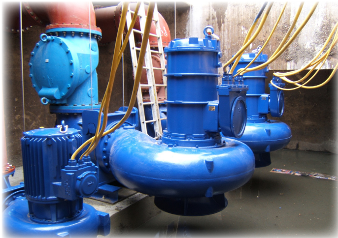
Two (2) large 24" discharge, 251 hp Submersible Pumps and one (1) 12" discharge, 80 hp on KSB guide cable system for a stormwater station.
