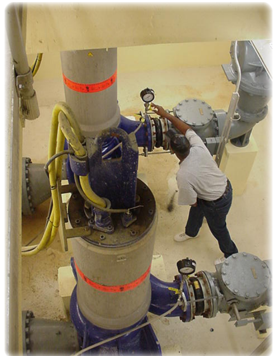
Three (3) 10" discharge, 194 hp closed-loop cooling dry-pit pumps with stainless steel Jacket in existing pumping station.
