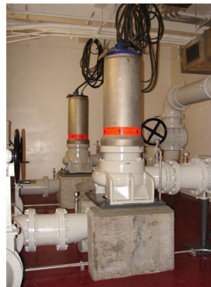
Three (3) 161 hp Dry-Pit Pumps with cooling jacket
