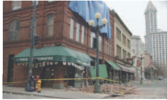
Seattle, WA, 03/05/01 -- Damage in Pioneer Square from the 02/28 earthquake. FEMA/Photo by: Liz Roll/FEMA News Photo
