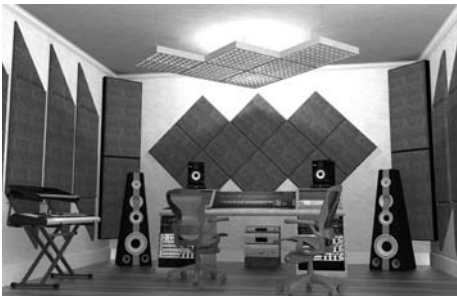
Six Radiator diffusers are bolted together and suspended above the mix position in a studio control room.
