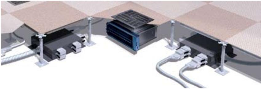
Control and power wiring are located under the floor, so they can be connected to the terminals via color coordinated plug-and-play connectors. Terminals can be added or removed to meet changing space configurations and loads, and control zones can be added or rearranged along with the furniture.
