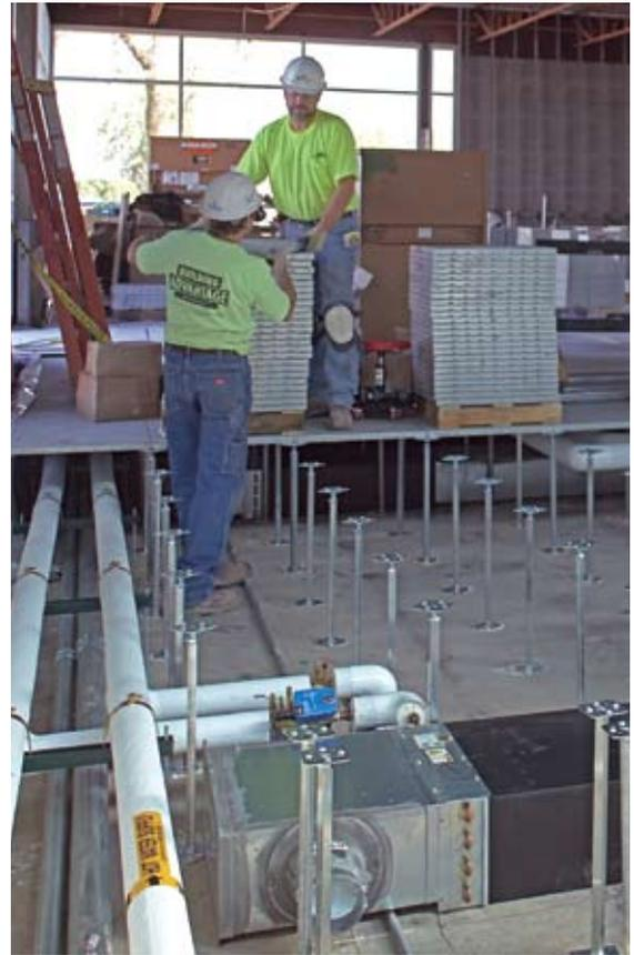
The FlexSys design provides easy access for utility service infrastructure and cabling during and after construction.
