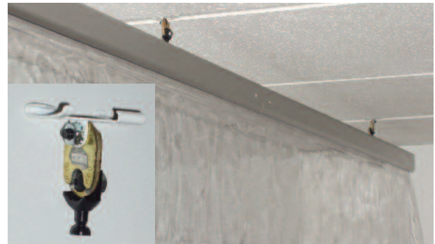
ContainAire Partition (close-up of fire suppression link)
