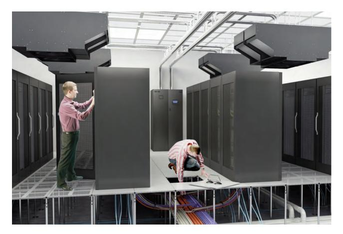
Overhead and above rack cooling systems have quickly become an accepted method for adding additional cooling capacity to high density rows of equipment. These systems are meant to compliment perimeter CRAC and CRAH unit designs to provide additional air delivery to the cold aisle. Refrigerant piping is routed overhead to a pumping unit which handles the exchanges from refrigerant to chilled water or outdoor air.
