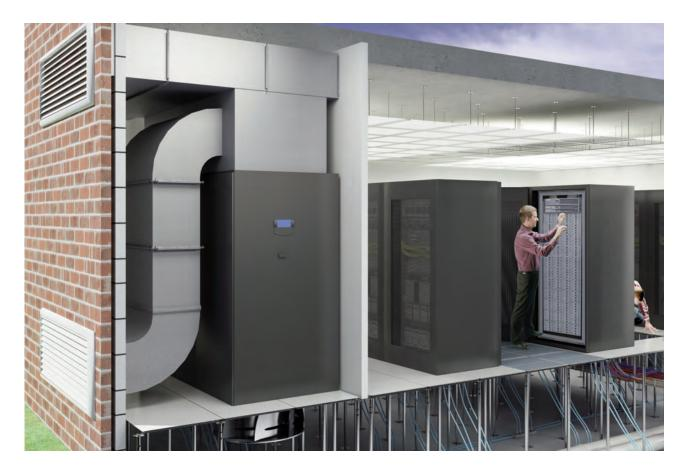
The use of air side economizing in the data center space has come into its own in recent years as one of the key ways to reduce the energy usage in the data center space. Historically deployed with containment methods and raised access floor, the overall impact on the data center energy bill is significant.
