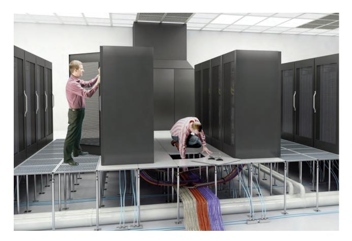
The most common data center design uses a perimeter CRAC or CRAH unit and raised floor to provide the ultimate in air flow distribution flexibility. The under floor plenum space allows the user to selectively distribute air at the volume required so equipment changes can be accommodated more cost effectively.
