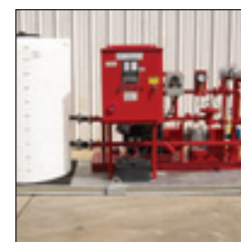
Diesel Pump Skids
