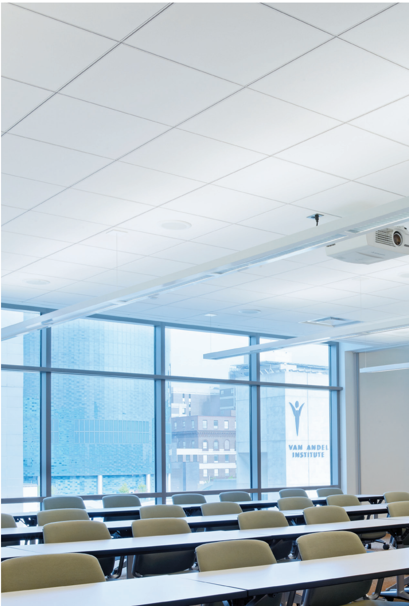
Ultima Ceiling-2-Ceiling Panels on Silhouette XL 1/4" Reveal Suspension System Secchia Center-Michigan State University College of Human Medicine, Grand Rapids, MI Ellenzweig, Cambridge, MA
