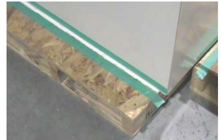
Figure 22: Horizontal seam filled completely with sealant
