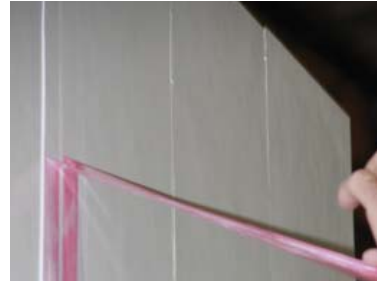
Figure 20: Removing Painter's tape
