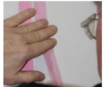
Figure 16: Applying the painter tape
