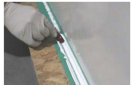
Figure 23: Horizontal finish with rounded corner
