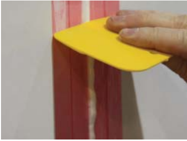
Figure 18: Removing excess sealant
