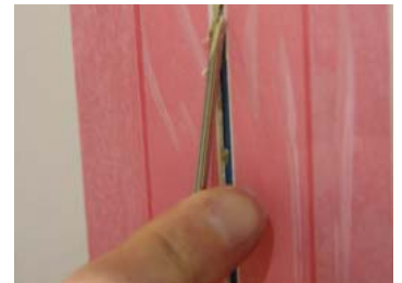
Figure 12: Remove excess adhesive
