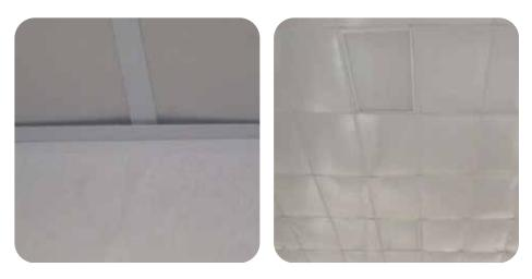
When FRP panels are placed in the grid, there will be a space due to the design of the grid. This space is accented, when using smooth panels.
