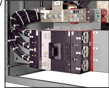
Fig. 13: Ground and neutral disconnect links
