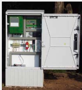
Control cabinet with station manager for automatic flow calculation
