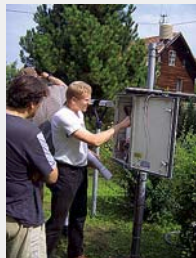
Inspection of the systems on location
