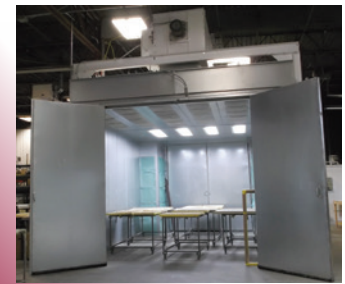
Batch Cure Chamber Interior
