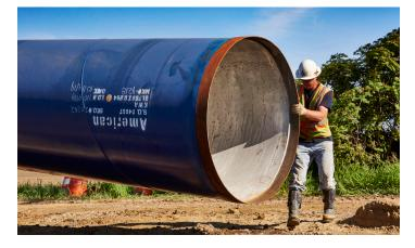
The conservative wall thickness recommended for the handling of steel pipe during the manufacturing, shipping and installation phases of a project is dependent on the type of coating and lining specified by the owner or owner's engineer. Steel pipe with flexible coatings and linings (e.g., polyurethanes, epoxies) should have a minimum diameter/wall thickness ratio (D/t) of 288. For conventional cement-mortar-lined steel water pipe, the recommended D/t ratio is no more than 240.
