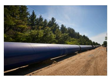
AMERICAN SpiralWeld Pipe supplies steel pipe for line work applications in diameters from 24 to 144 inches and joint lengths up to 50 feet. Line work typically includes:
