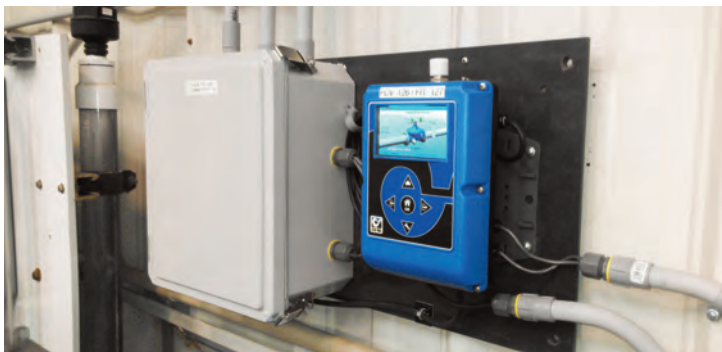
Typical installation with mounting bracket
