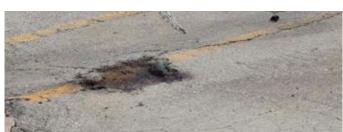
**Cleans** – Dust and debris is blown from the pothole by a high velocity blower. The Operator is located in the cab eliminating being exposed to traffic and reducing the risk of potential personal injury.
