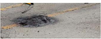
**Tacks** – Asphalt emulsion is sprayed to seal the surface and create a binder for the repair. A nozzle tilt allows for more efficient movement of rock when cleaning the repair and reduces rock bounce.
