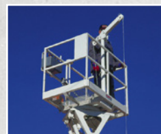
MATERIAL HANDLING IN WORK PLATFORM
