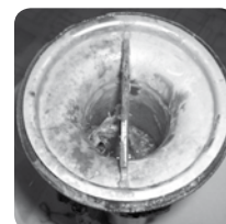
Old water trap after 2 months
