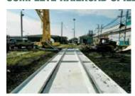
ENPAC's railcar track pans are a heavy-duty modular fiberglass system designed specifically for railroad spill containment. Contains small leaks as well as large spills without interfering with normal railcar operations. Simply connect multiple units to provide spill containment for hundreds of feet of railcar. Plumb drains to a remote
