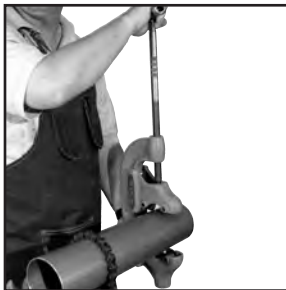
Figure 1: Cut tube to desired length using s tube cutter
