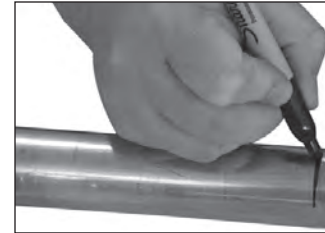
Figure 3 — Marking for Insertion Depth
