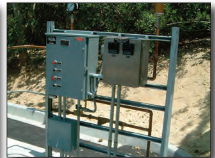
Remote SCADA control
