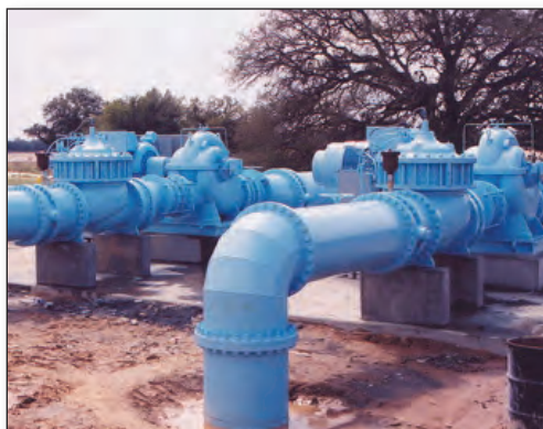
30-Inch Pump Control Valves
