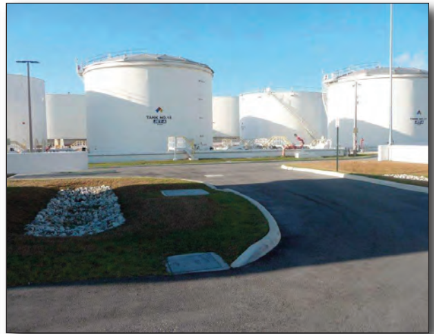
Commercial Aviation Fueling System - Fuel Storage Tanks
