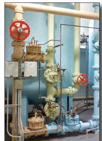
Multiple Valves in Industrial Application
