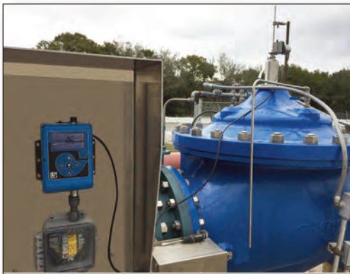
Aquifer Storage Recovery System with 131 Series Electronic Valve & VC-22D Electronic Valve Controller for Reclaimed Water
