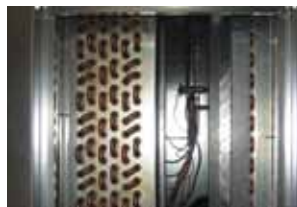
PDX & Hot Gas Reheat Coils
