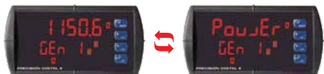
Upper line toggles between 1150.6 and Apparent Power and the lower line displays Gen 1
