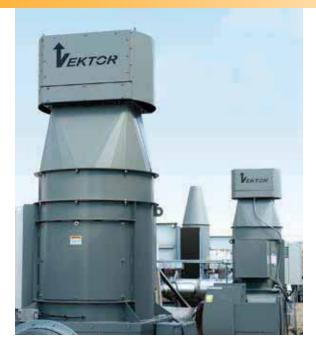
Greenheck has the most extensive line of laboratory exhaust systems in the industry. The main objective of a laboratory exhaust system is to remove hazardous or noxious fumes from a laboratory, dilute the fumes as much as possible and expel them from the laboratory building preventing contamination of the roof areas and re-entrainment into building make-up air systems.
