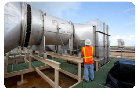
Paint Booth Exhaust
