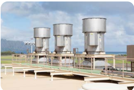
Paint Booth Exhaust
