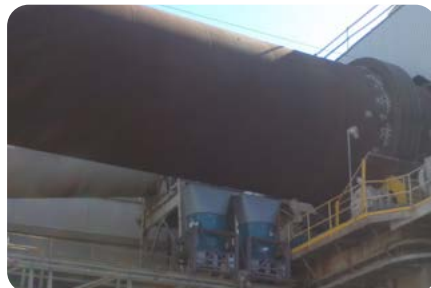
Cement Kiln Cooling
