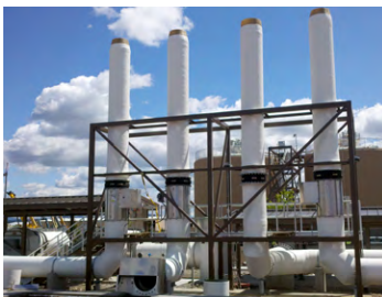
Biofilter Exhaust
