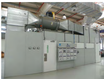
Paint Spray Booth
