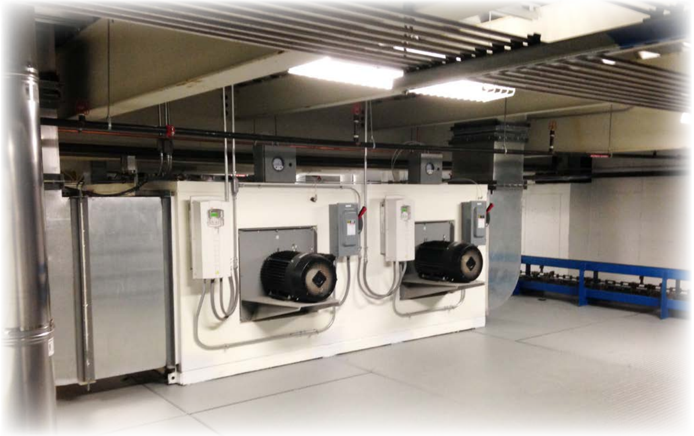
Recirculation Fans in Paint Finishing System
