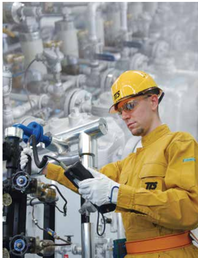
▲ Figure 1. The steam-trap survey is the key component of a steam-trap management program. However, a plant should not jump into performing the survey without proper planning and preparation.
