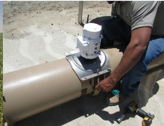
FlowConnect is a built-in solution for data collection and transmission of flow data from McCrometer's McPropeller and Water Specialties Propeller Meters. FlowConnect's innovative design eliminates the need for cables, pole mounting and other hardware, setting it apart from traditional telemetry systems.
