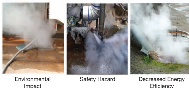
▲ Figure 3. There are many places in plants where condensate is not recovered. This can create a negative environmental impact, pose a safety risk, and reduce the energy efficiency of the plant.
