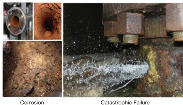
▲ Figure 4. Corroded pipes in condensate return systems are more susceptible to leaking and catastrophic failure, especially if they are subject to shock from water hammer.
