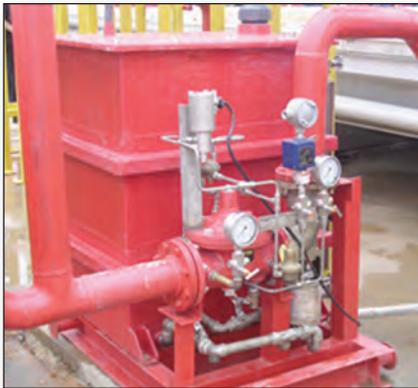
The DIFFS utilizes the Cla-Val Model 134-60 Automatic Deluge Control Valve to quickly dispense foam or water, extinguishing flames in less than 15 seconds.
