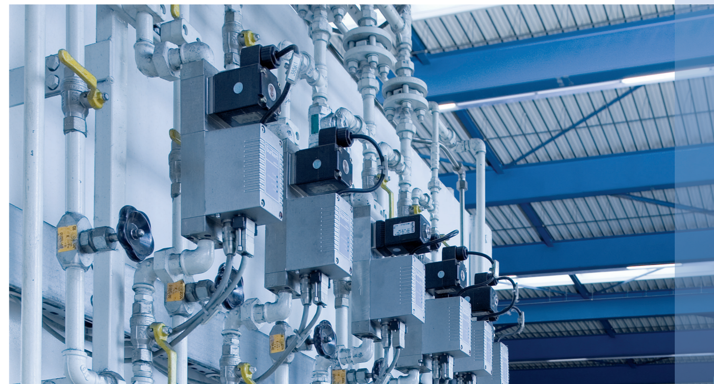
The MFCs provide defined atmospheres to guarantee reproducible processes. The atmosphere volume can range from a specific point on a weld seam to the chamber volume of a hardening furnace.
