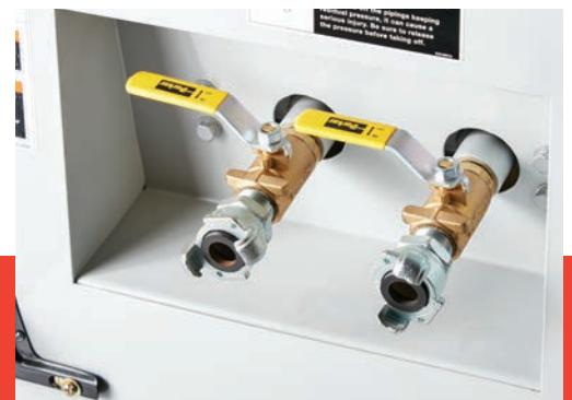
Two 3/4" NPT air service connections
