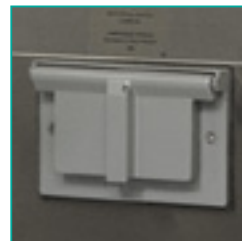
Duplex and/or GFI Outlets
