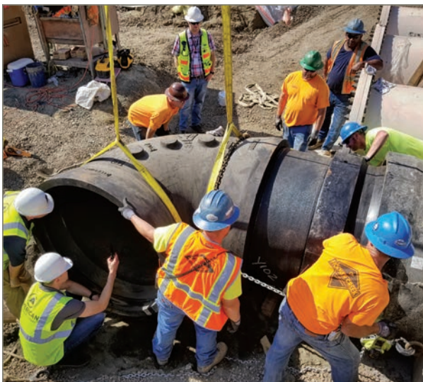
AMERICAN Flex-Lok wall pipe in combination with Flex-Ring pipe and fittings is an excellent choice in seismic applications to allow for extreme movement.
