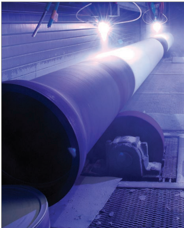
Metallized arc-spray application of zinc coating.
