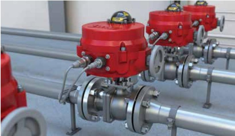
*Typical installation of Series 70 DeviceNet Actuator*
