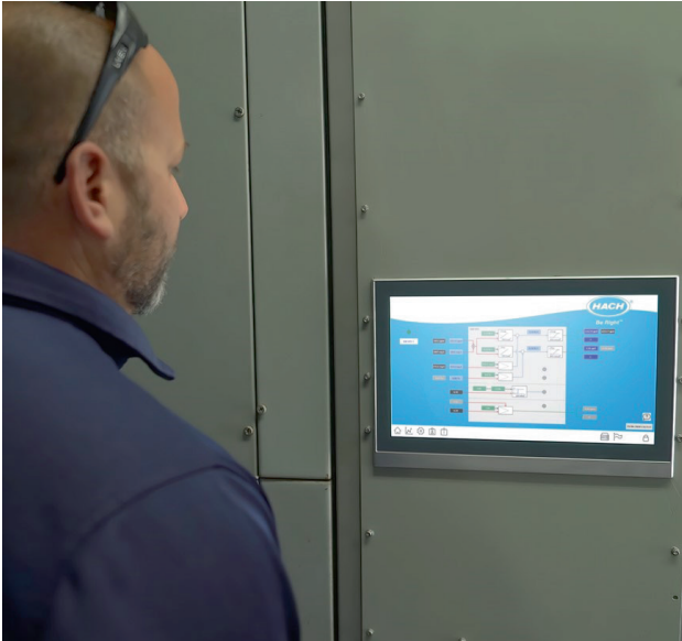
Examples of a typical RTC installation and RTC-COAG user interface screens. All settings, validity and fallback strategies are configured through the touchscreen and can be password protected.
